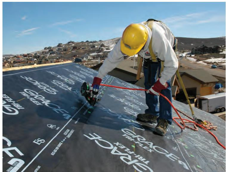
**It's more durable**—Grace Tri-Flex can be left exposed for up to 6 months. It doesn't dry out or rot at high temperatures. It doesn't crack or become brittle at low temperatures.
