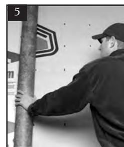
1. With the wall on the ground, start at one corner, allowing an extra 12" (304 mm) flap for the corner and align the guide marks on the Typar with the studs.
